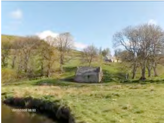
Fig. 4 site of turbine house to right of old mill building, Don and site of out fall in foreground
