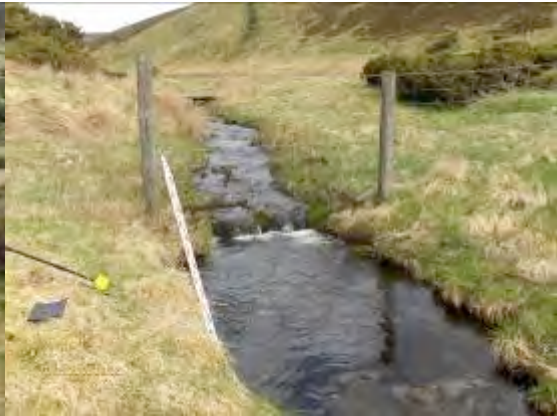
Fig. 3 Burn at site of intake weir
